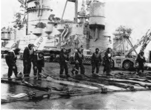
Rigging the barrier
